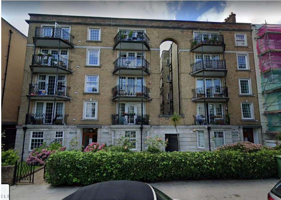
Plate 1: East facing (front) elevation of 35 Belsize Park.
