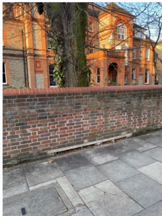
Lintel to wall accommodating tree T1
