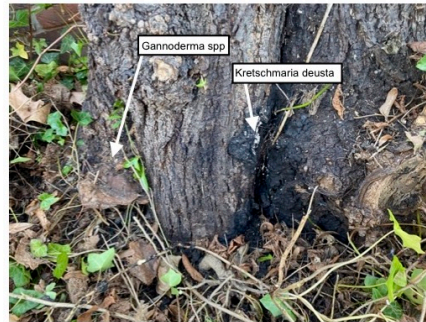
Kretschmaria deusta fruiting bodies extending to 300mm height and Ganoderma to north at base of tree
