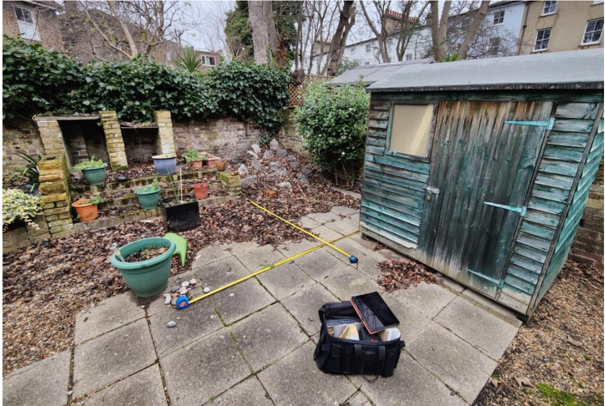
Existing timber building to be removed.
