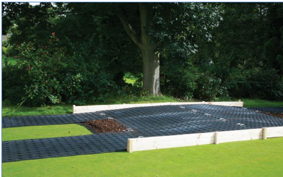
Green-Tek Ground Guards showing geotextile membrane, 100 mm of woodchip with panels above protect tree roots
