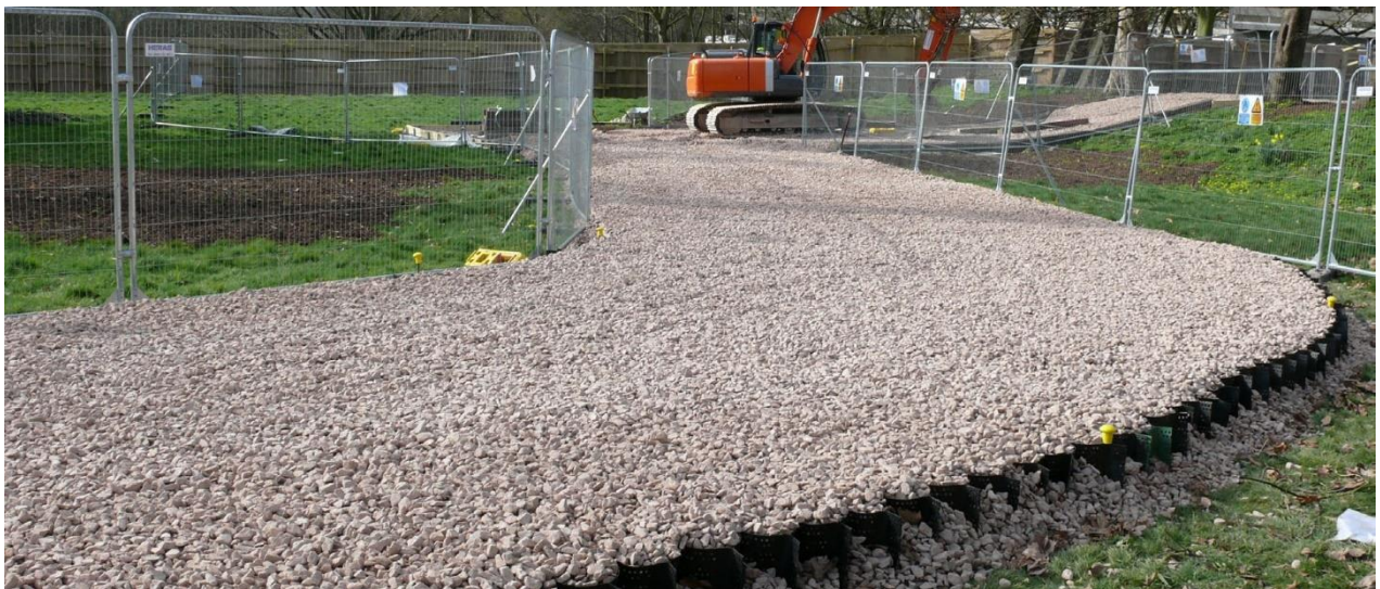
Images of cellular confinement systems and edging detail
