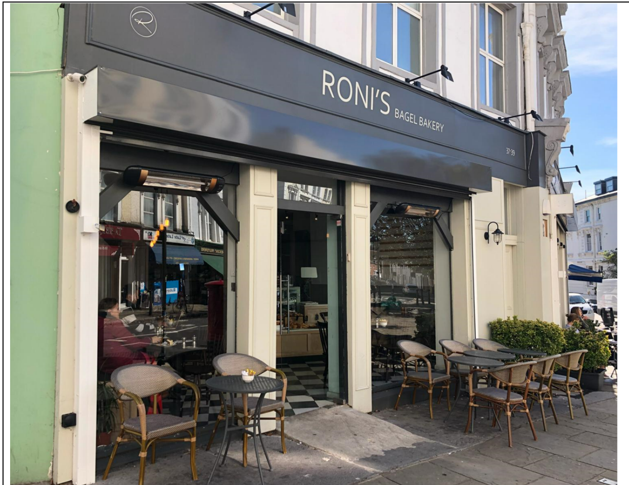
Image 1: External shutter housing box, shutter frame, external heaters (Sept 2018)
