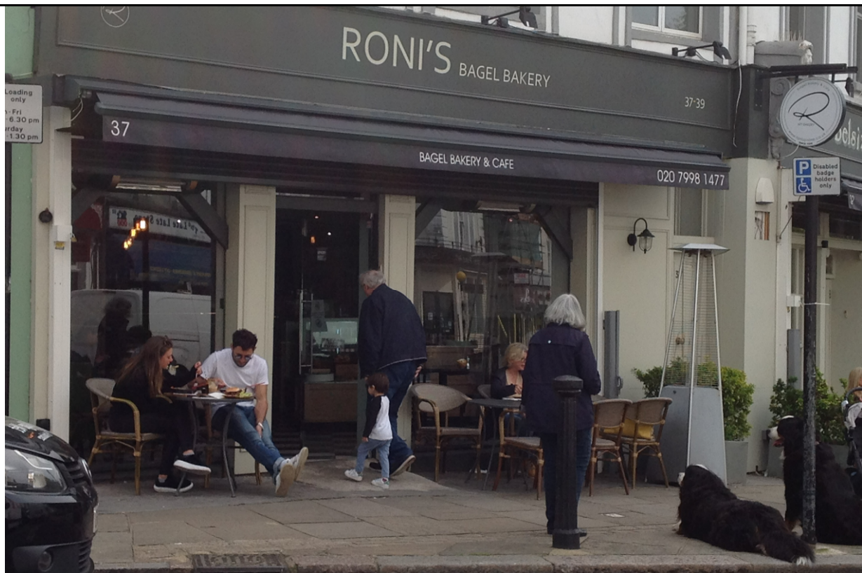
Image 2: External shutter, housing frame with awning above, external heaters (June 2019)
