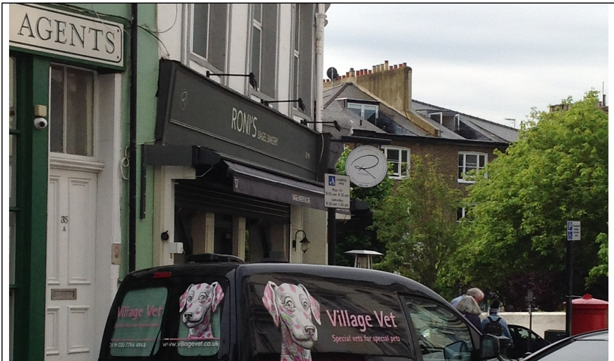
Image 3: projection of awning housing and projecting sign (June 2019)
