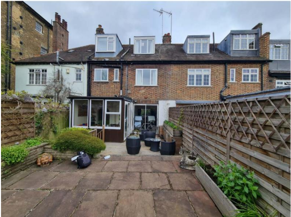
5. Photo showing rear elevation of application site and adjoining properties
