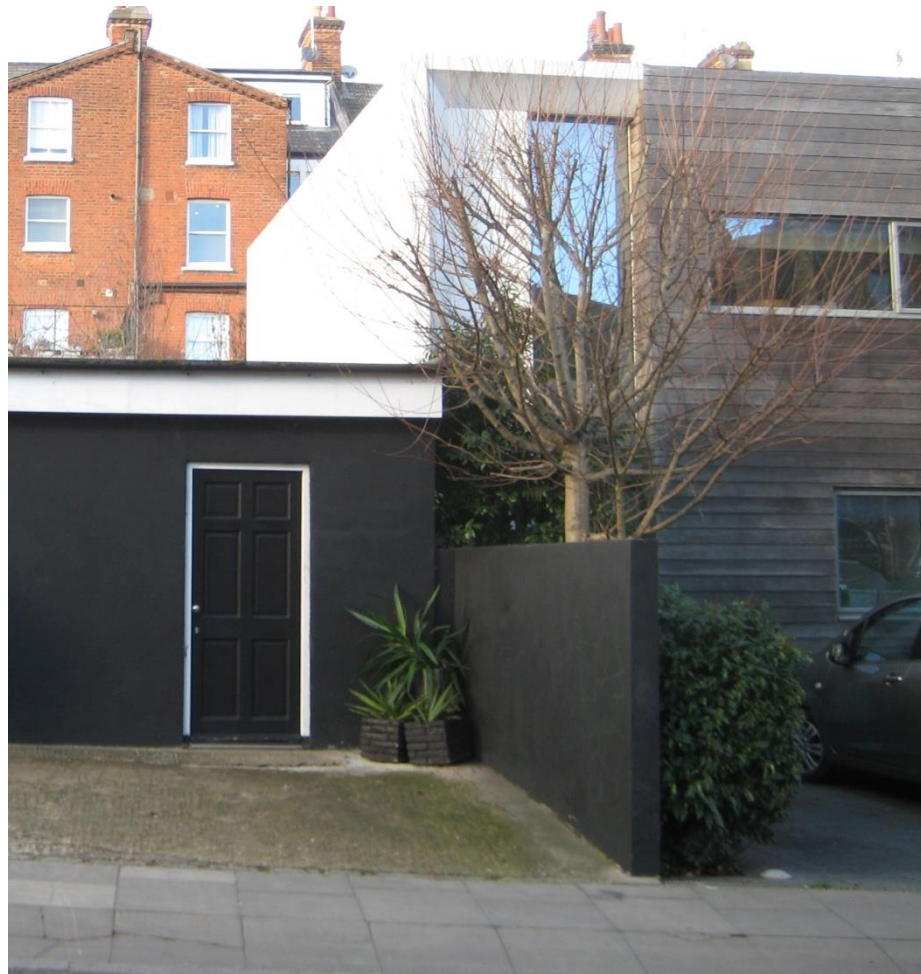
Fig 6 – Existing hard standing within the RPA of T4 ( Acer spp ). This is retained for the duration of all construction works before being removed by hand and soft landscaped.
