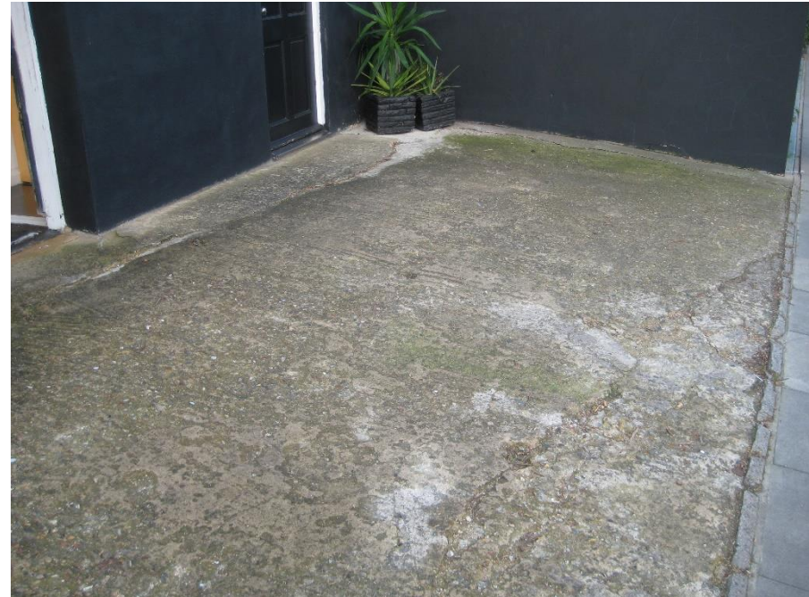
Image 3 –Existing hard standing within the RPA of T4. This should be retained during the works and removed only after all the main construction activity is complete.
