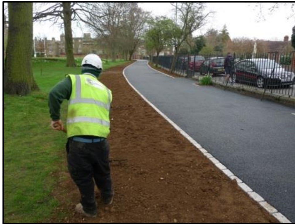
Fig 13 – All 'making good' topsoil will be BS3882 compliant and raked out by hand to no greater depth than 100mm
