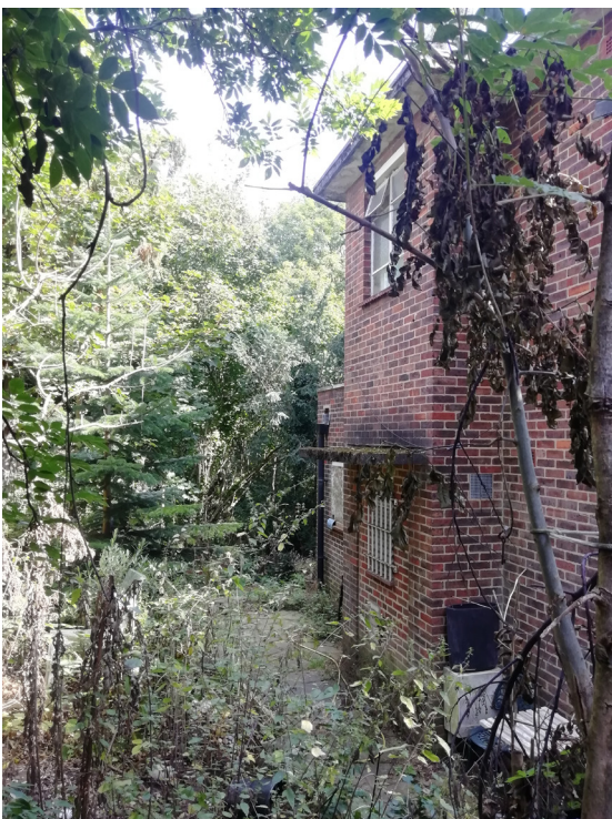
3. Existing front entrance (now blocked up)
