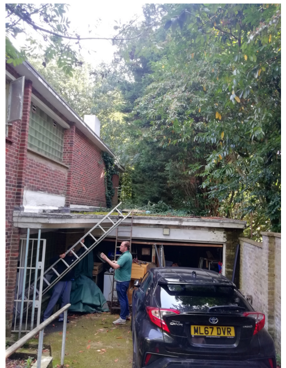
4. Existing double garage and side entrance
