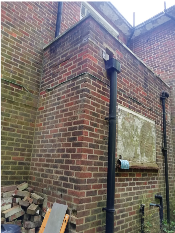
7, 8 and 9. Existing brickwork
