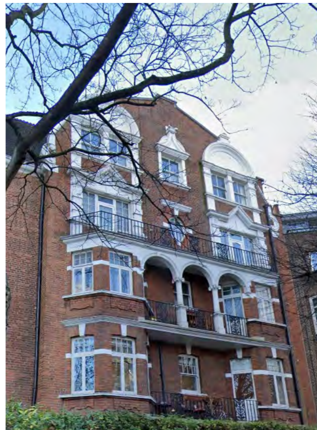
Kings Gardens mansion block to the South
