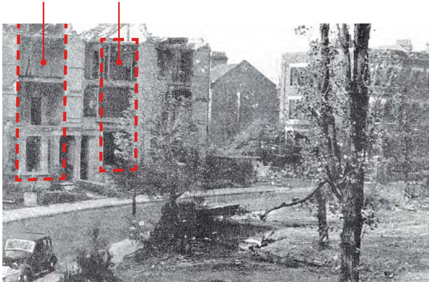
View of Gascony Avenue / West End Lane showing bomb damage
