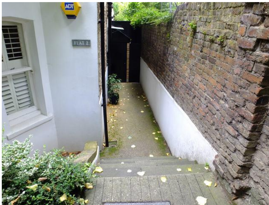
Image 12 Steps leading down to the entrance, with some space for materials.
