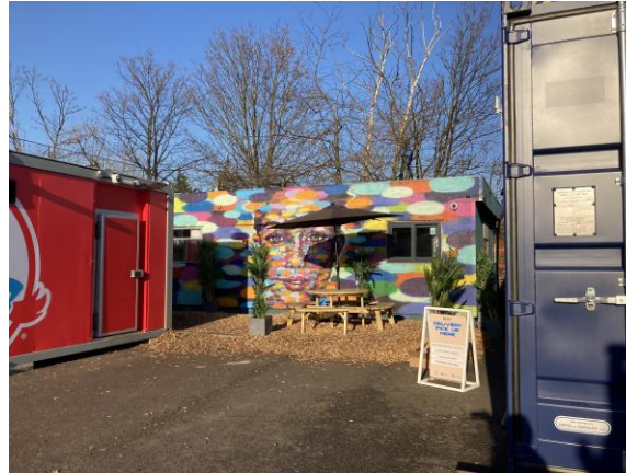
Photo 2: Example image of three of the buildings on site.
