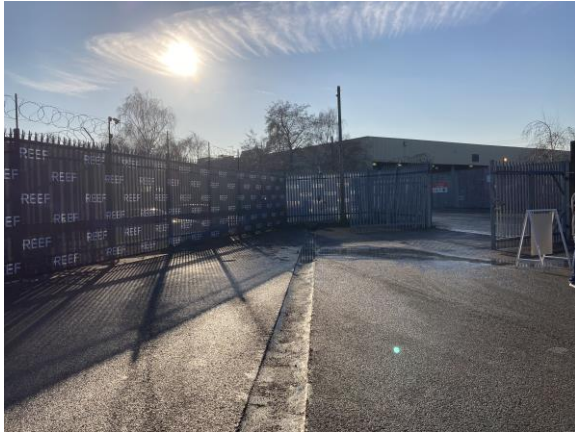
Photo 1: Hardstanding and fence on site.
