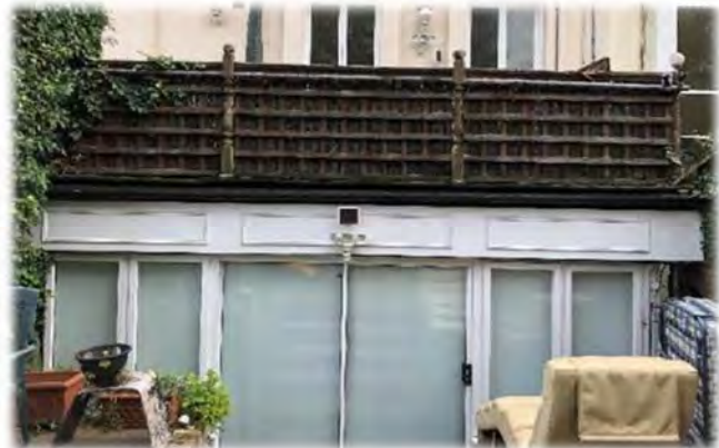
BASEMENT LEVEL CONSERVATORY
