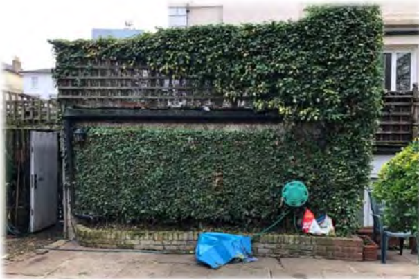
GROUND FLOOR GARAGE
