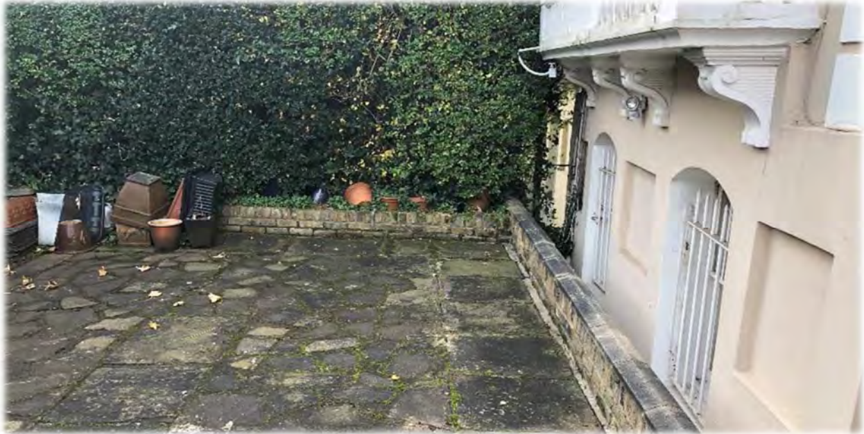
EXISTING FRONT PATIO / GARDEN
