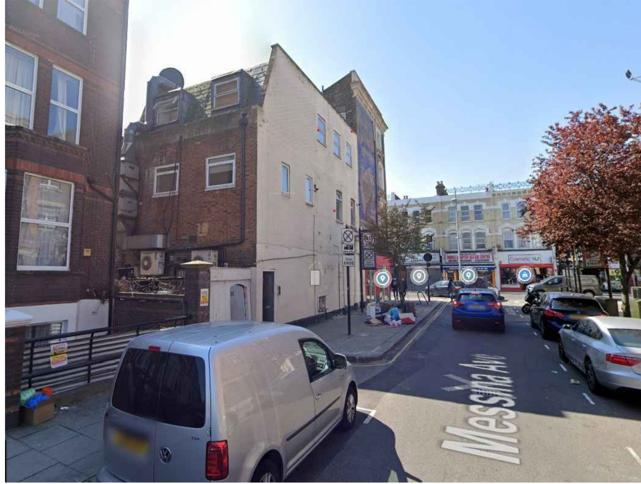
01 EXISTING STREET VIEW A
