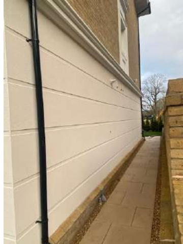
Example of rendered wall with full length straight grooves.
