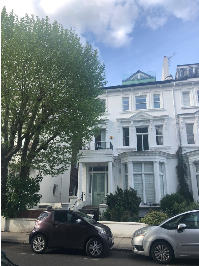
Front elevation of 22 Belsize Park Gardens showing the front roof balcony
