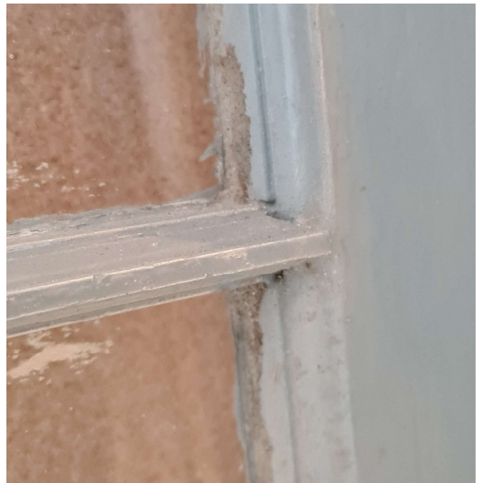
5.08 Ovolo and Fillet glazing bar detail
