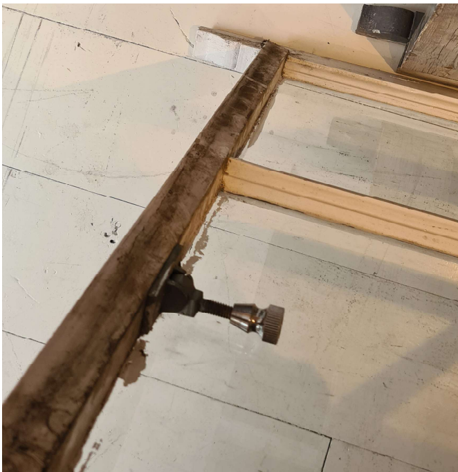
5.07 Hardware/fitings in good condition throughout
