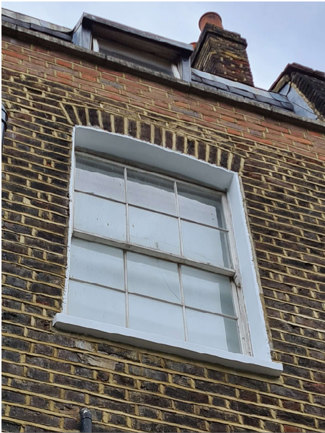
5.05 Existing second floor rear window for reference
