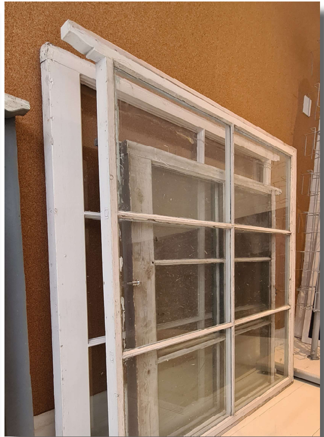
5.06 Reusable sashes removed for inspection
