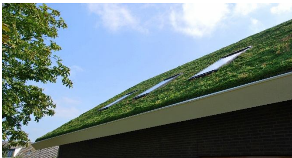
Example; grey timber clad (below) & of a green pitched roof (above)
