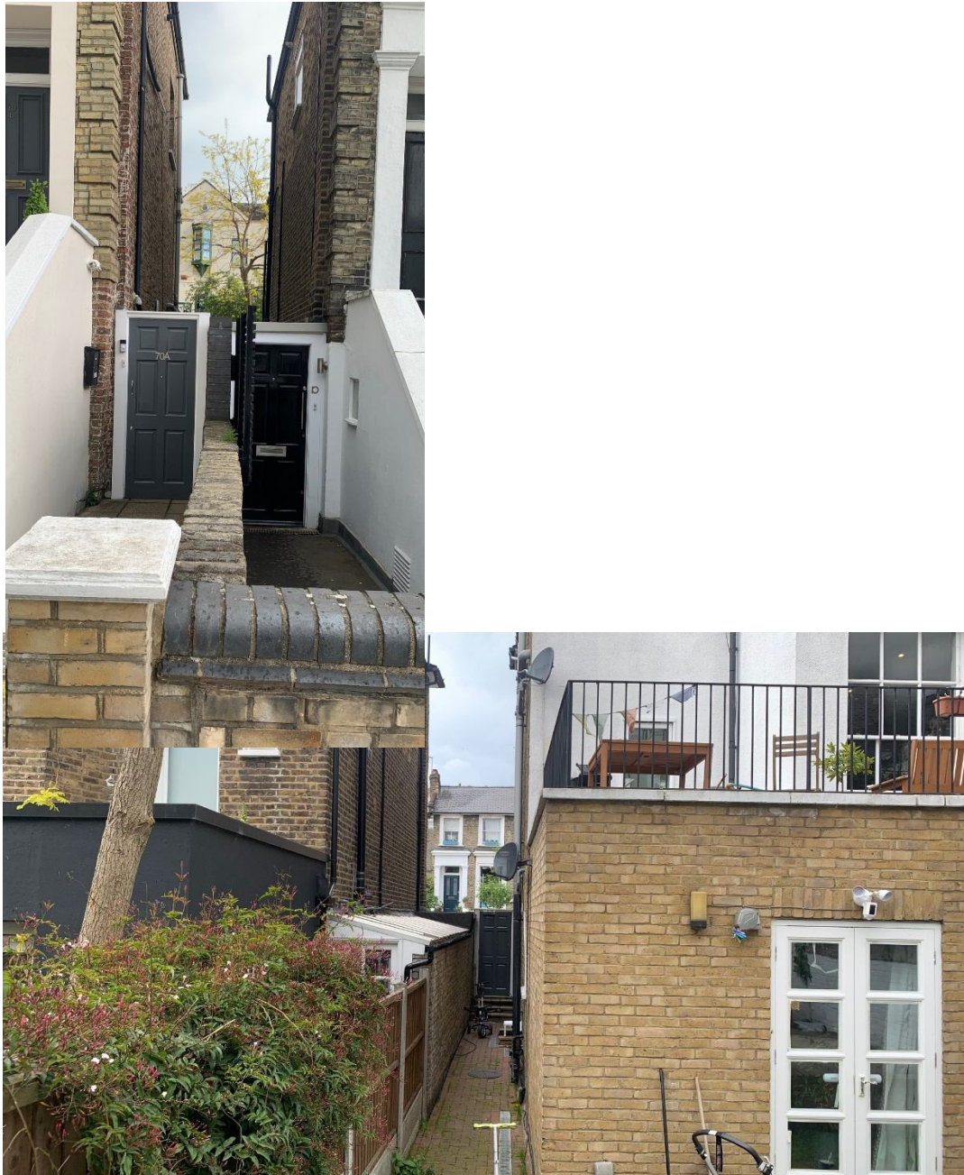
Photos showing entrance, & side (lower ground level) where permission to extend has already been agreed
