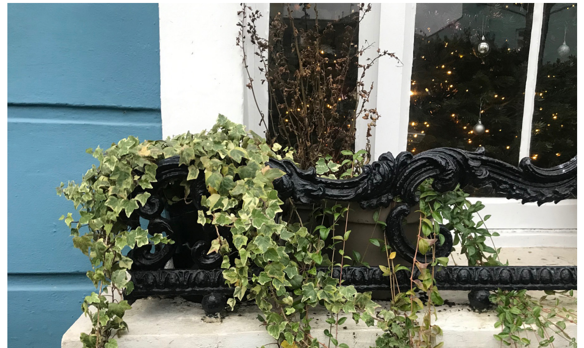
Black cast iron window guards
