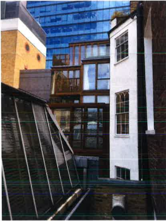
View east showing existing Upper Floor terraces at No. 29 Percy Street
