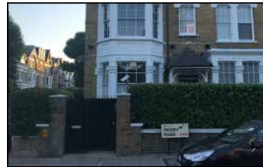
02 Priory Rd Site Elevation view
