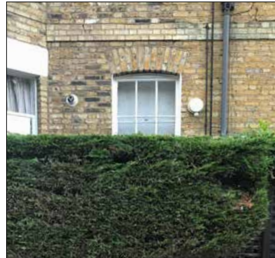
02 View from Cleve Road of the window opening proposed for replacement.
