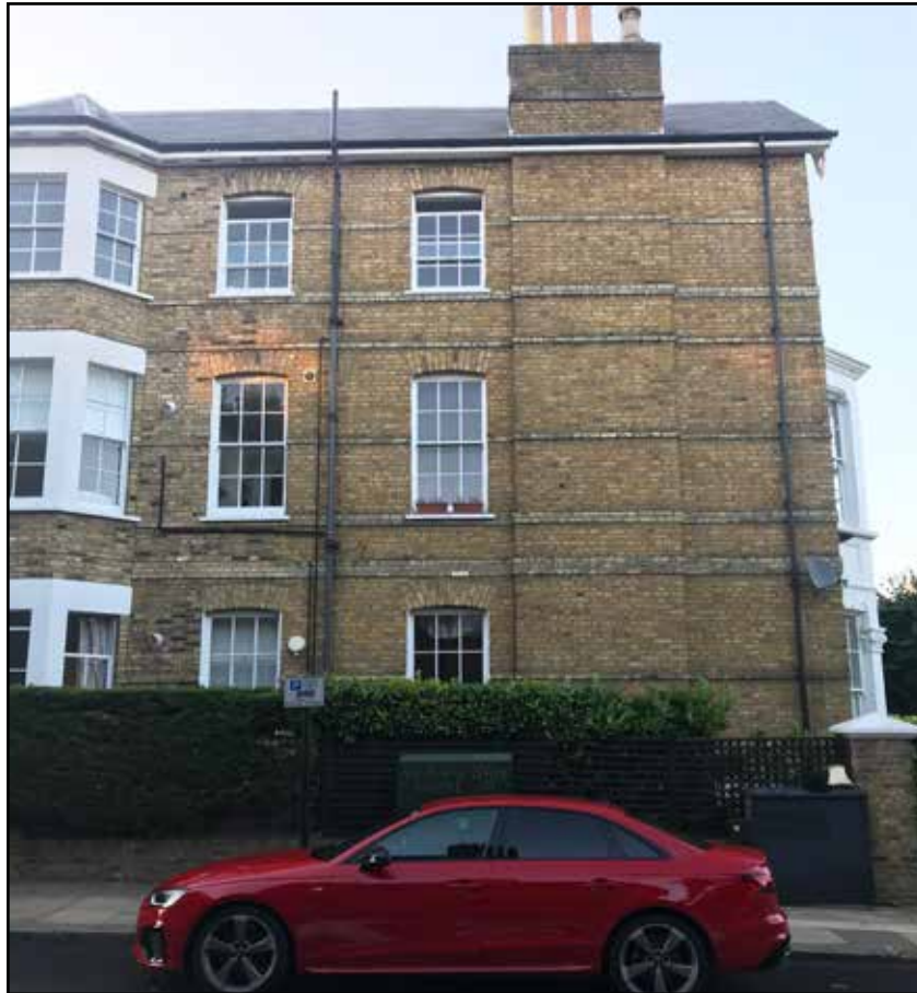
01 View of the side elevation from Cleve Rd. Note: The application site relates to the Ground Floor of Flat A only.
