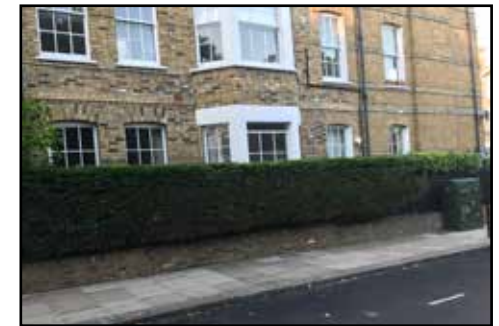
03 Cleve Rd Site Elevation view showing high level hedge part concealing the Ground Floor fenestration.
