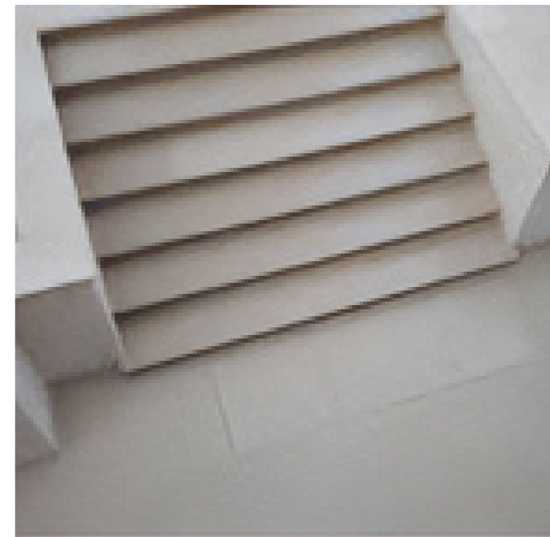
Portland stone steps
