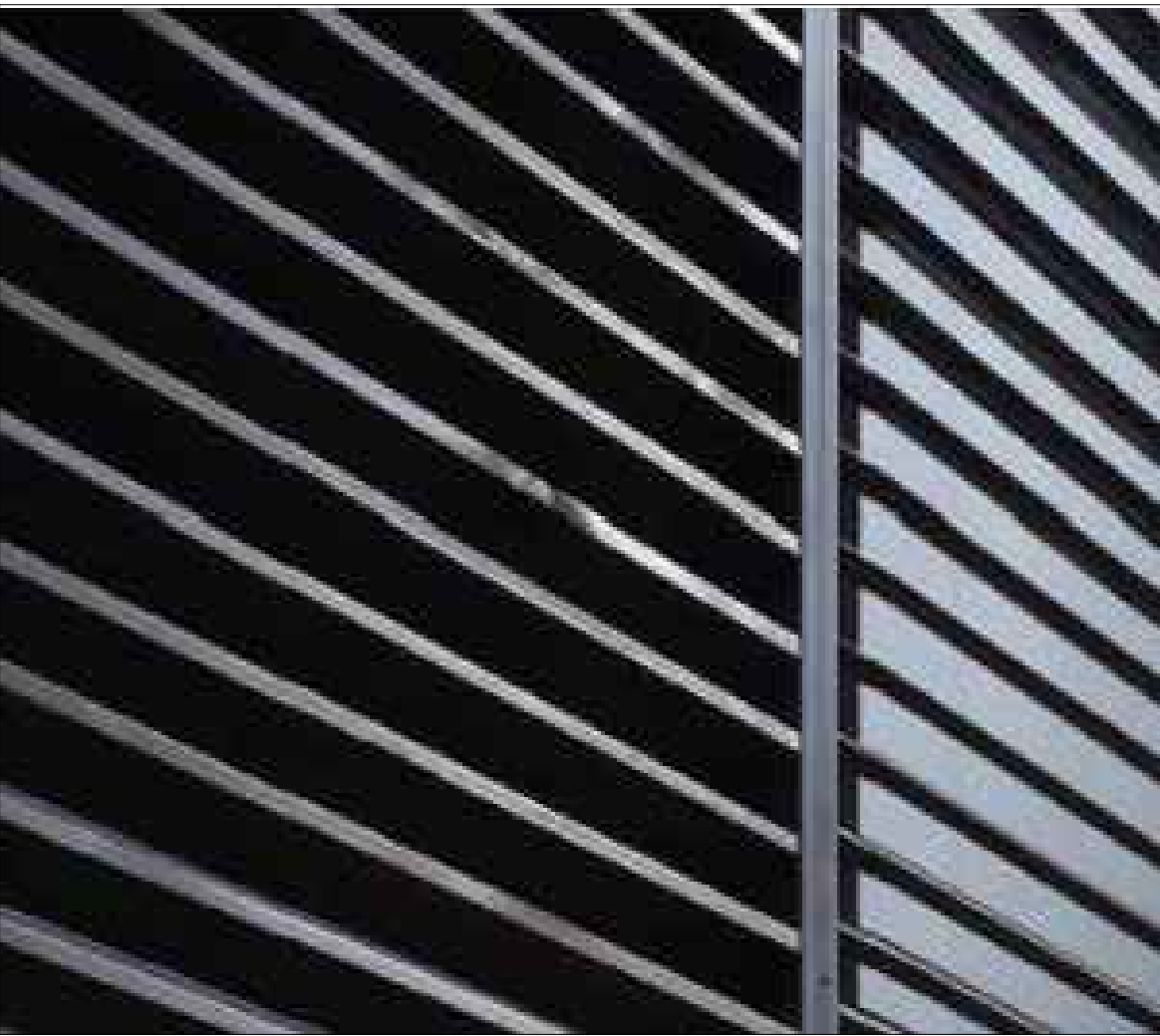
2 Ventilation louvre panels above entrance doors
