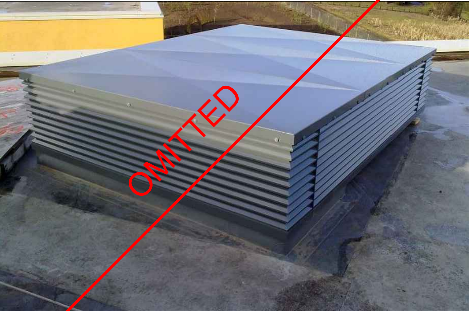
3 Louvered Penthouse Vent for AHU Exhaust
