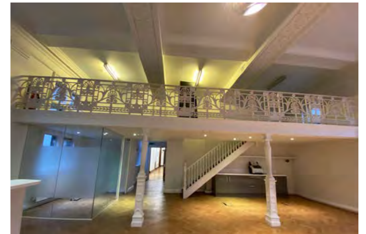
Figure 4.23 View of existing mezzanine on second floor, Library
