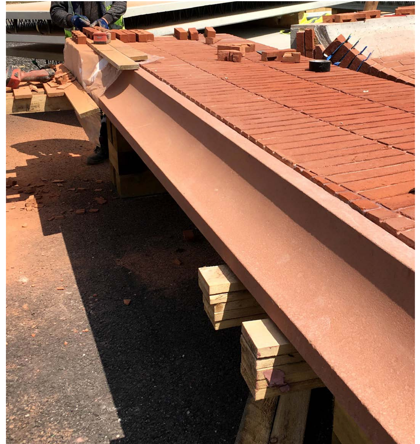
Figure 8: Red Recon Stone Corner Piece Fitted Into An Arch Panel
