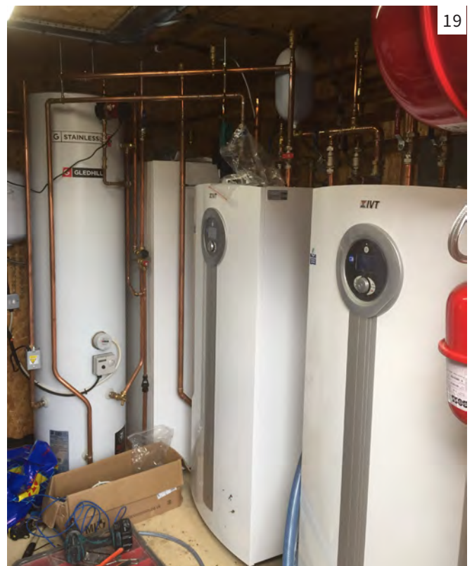
18,19 Plant rooms with large heat pump installations.
