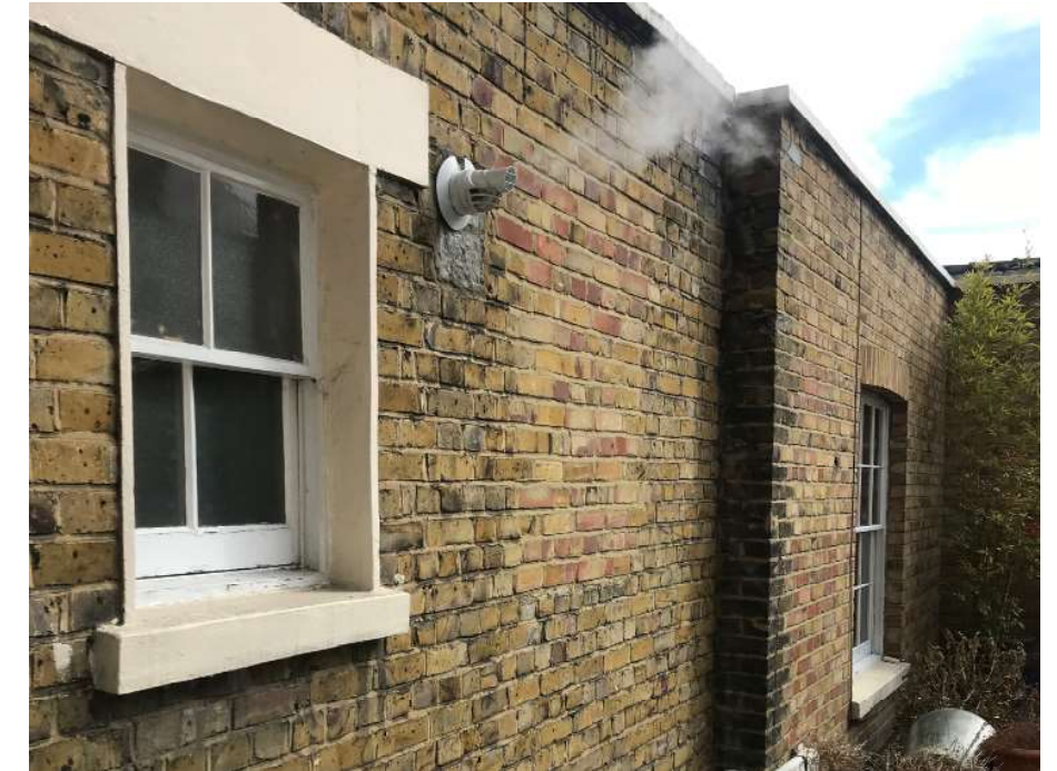
Existing sash window to be enlarged and reinstate window next to it.
