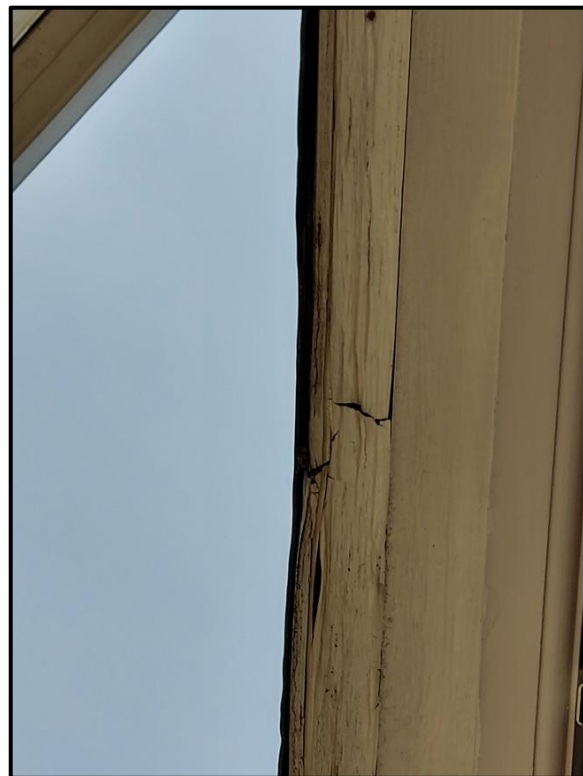
Figures 6, 7, 8 & 9: Photographs showing the poor condition of the top floor windows that will require replacement
