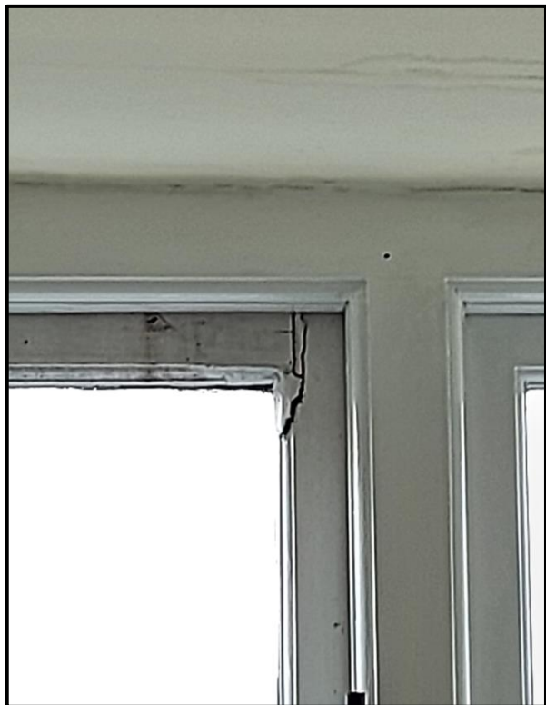
Figures 10, 11, 12 & 13: Photographs showing the poor condition of the top floor windows that will require replacement
