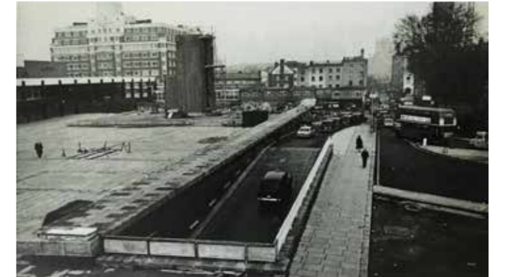
Figure 3.14 Looking east towards Euston House across Euston Piazza in the 1960s, during construction of the Seifert office development
