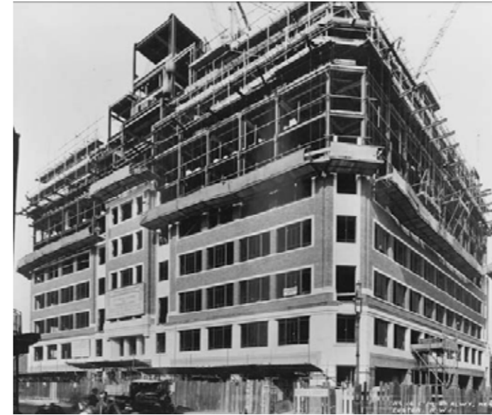
Figure 3.11 Euston House under construction, 1933-34
