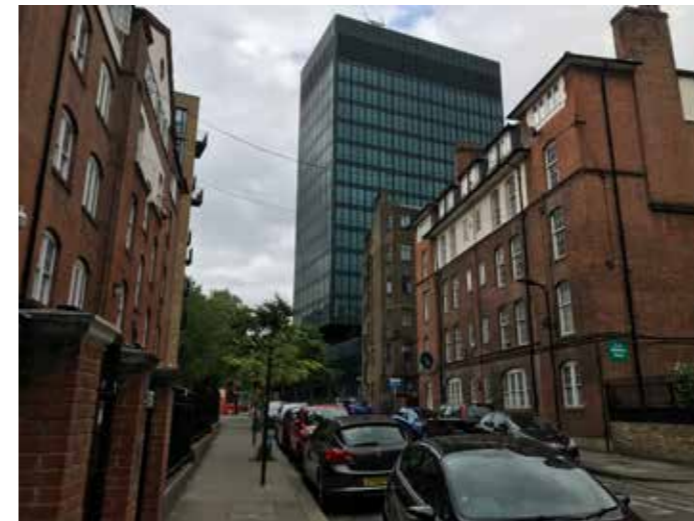
Figure 4.11 Seymour House and Wellesley House, with Grafton Chambers behind, on Churchway
