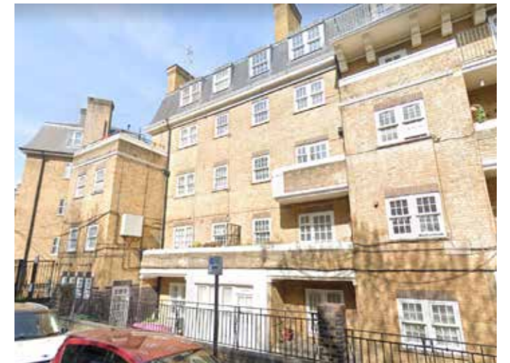
Figure 4.12 The St Pancras Housing Association Estate, Doric Way
