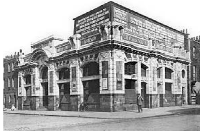
Figure 3.8 Euston Underground Railway entrance, c1920, at the corner of Eversholt Street and Doric Way.
