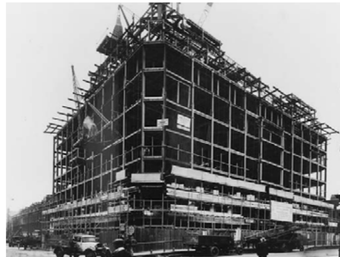
Figure 3.10 Euston House under construction, 1933-34
