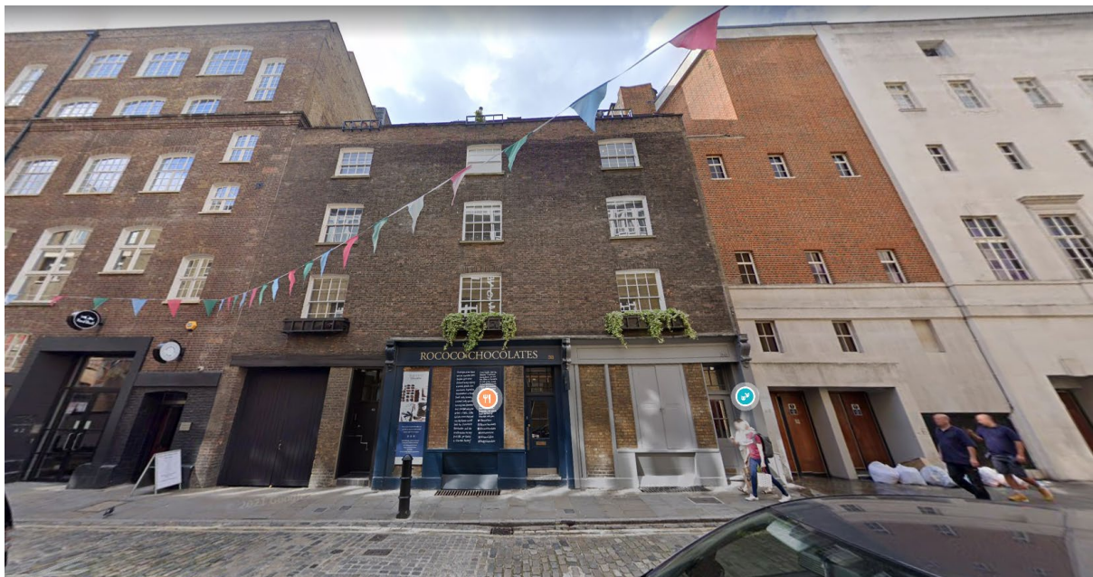
Flat A, No. 40 Earlham Street, London WC2
