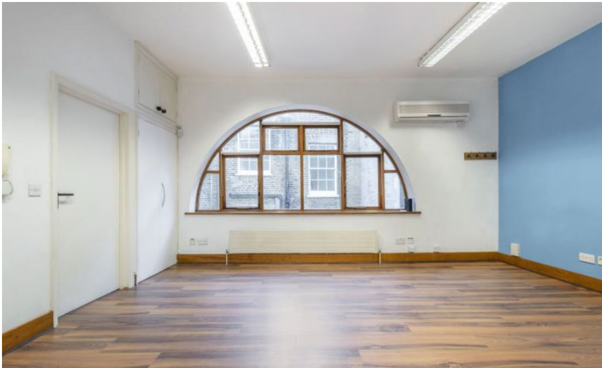
3 rd Floor – existing Diocletian window – glazing to be replaced and the ceiling to be dropped.
