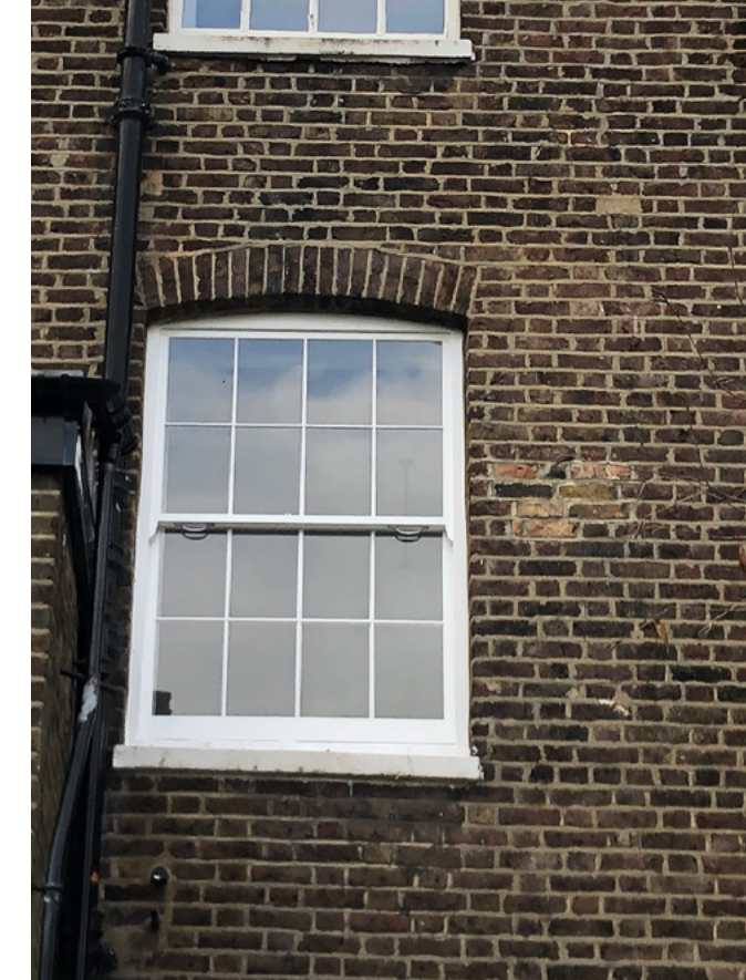
Images of rear exterior and existing pointing conditions - poor, weathered and dirty.
