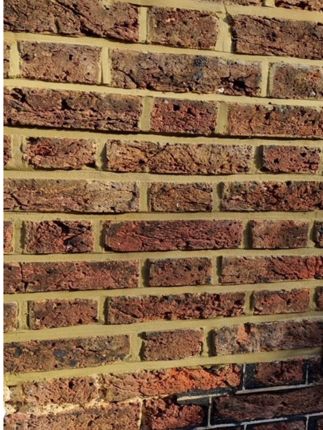
Sample of repointing on front facade with weatherstruck repointing - this is to be repaired using the following method statement and recessed pointing will be employed.
