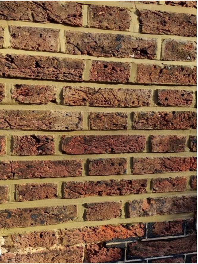
Sample of repointing on front facade with weatherstruck repointing - this is to be repaired using the following method statement.
