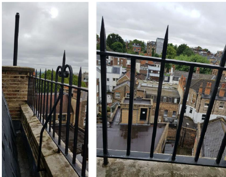
Figure 4: Steel powder coated railings
