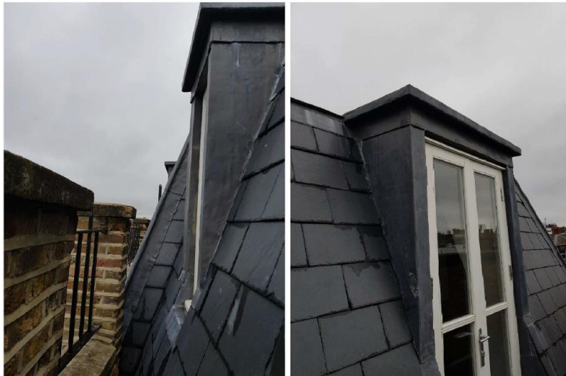
Figure 3: Lead clad dormers with painted timber windows
