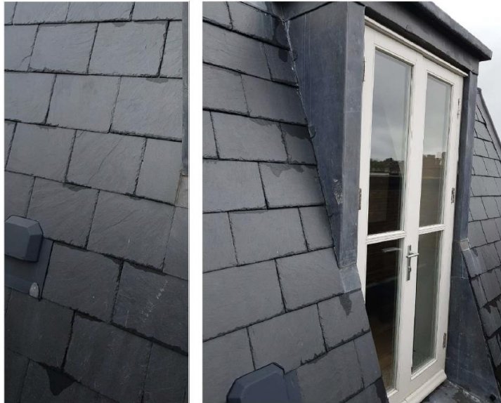
Figure 2: Mansard roof finish – man-made slate with lead cheek dormers
