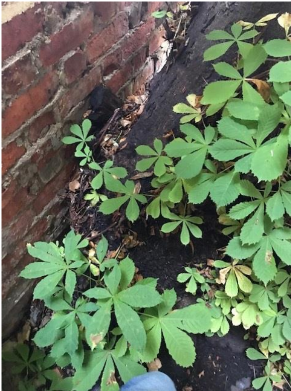
Photograph 1: Showing contact with rear boundary wall.
