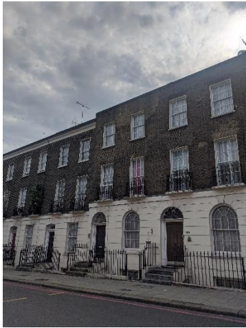
Figure 2: Existing painted section on front elevation
