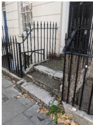
Figure 4: Existing front entrance steps
