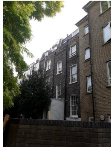
Figure 3: Existing brickwork sections on rear elevation
