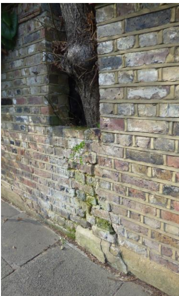
1: Wall in front of T1
