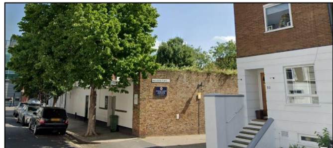
Figure 3: Rear Boundary to Waterside Place
