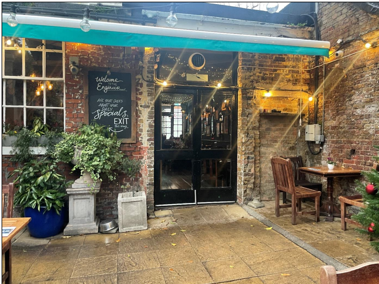
Figure 9: Modern Rear Entrance Door In Late 19 th Century Altered Elevation With Window In Mid-18 th Century Building Adjacent.
