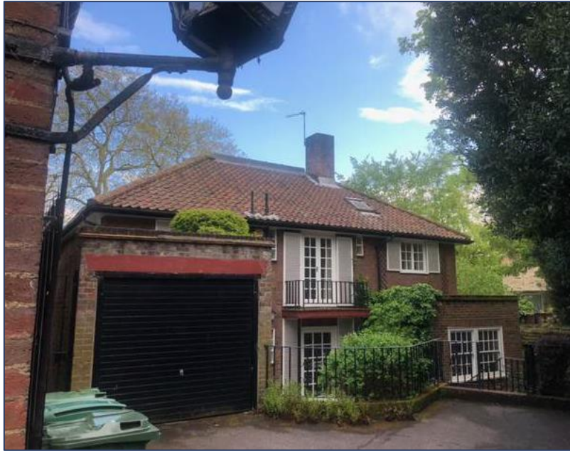
Figure 4 - View of the front of the property, showing the garage to the left of the image
