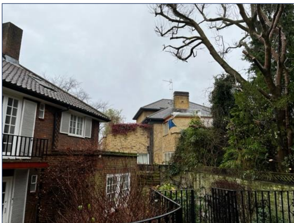
Figure 11- View from the appeal property to the under construction extension above the eaves height at the neighbouring 18 Frogmal Way
