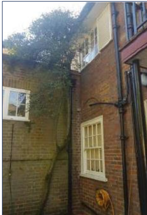
Figure 12- Existing front entrance area
