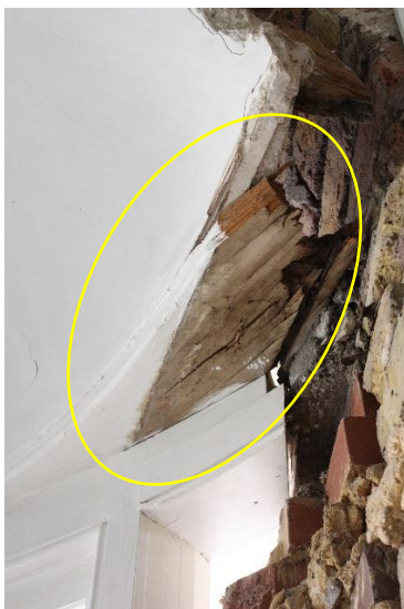
Photo 4. Rot in eastern end of lintel.
