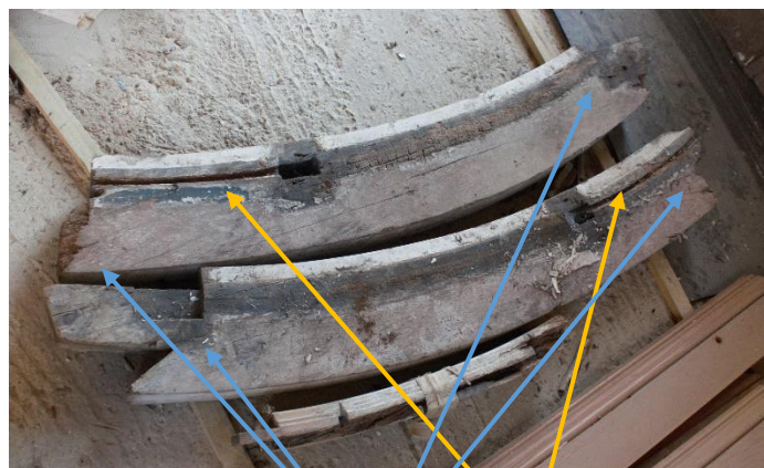
Photo 5. Two part oak sill, note groove for weather strip in central section, rot at both ends and middle.
