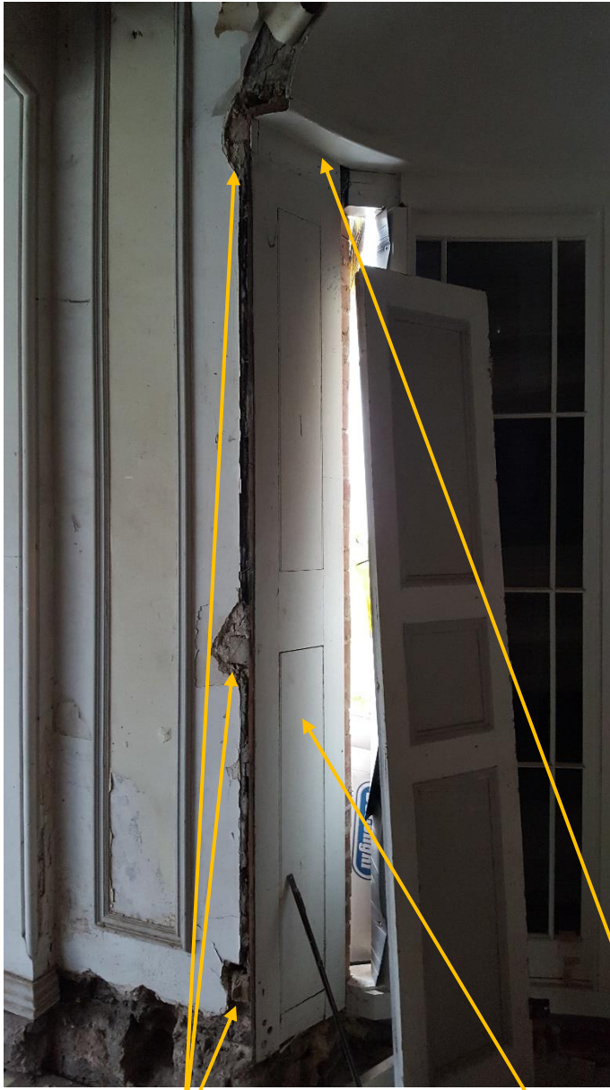
Photo 6. Note grounds set in wall, shutter box liner and soffit still in situ.
