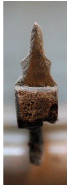
Photo 3. Profile of glazing bar
