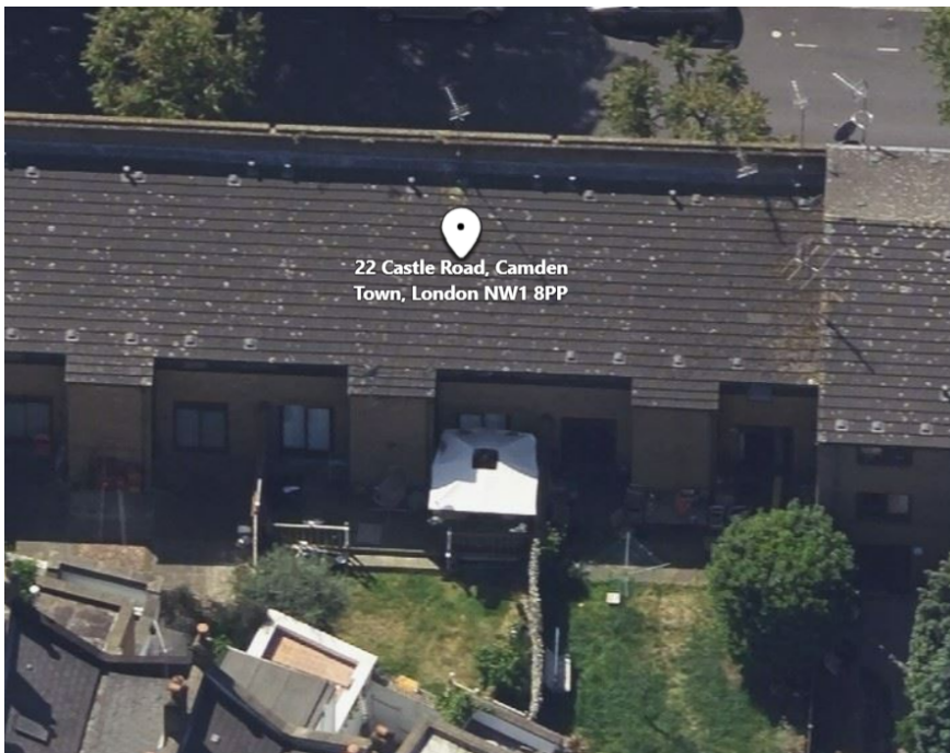
View 2 – aerial view showing rear roofslope of application site
