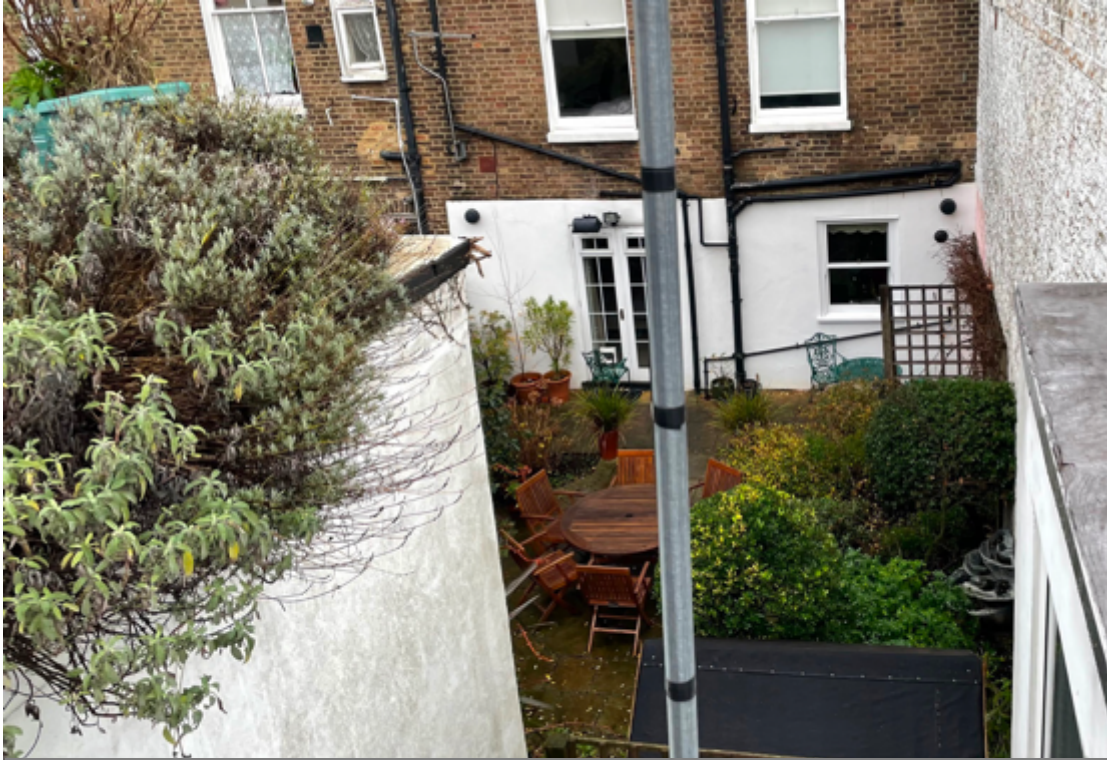
View looking into rear of No. 5 Belsize Crescent from 1 st floor of the development site.
