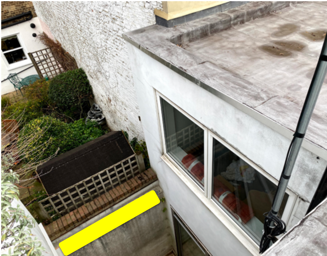
View looking into rear of No. 5 Belsize Crescent from development site. The yellow box indicates the siting of the proposed high-level windows.
