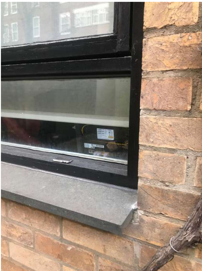
Detail of a typical rear window to be replaced. Existing cill to be retained.
