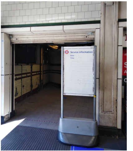
Existing View into unit : Roller shutter open
