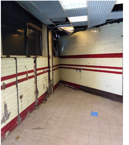
Internal View into shop: Windows blocked off internally with black paint/vinyl/board
