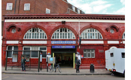
External Street View to Station: Windows blocked off, creating lack of visibility into the unit from street level
