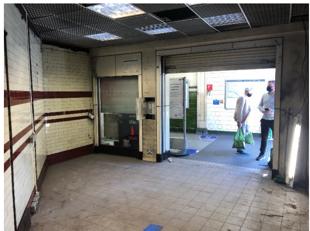
Inside of the Unit
