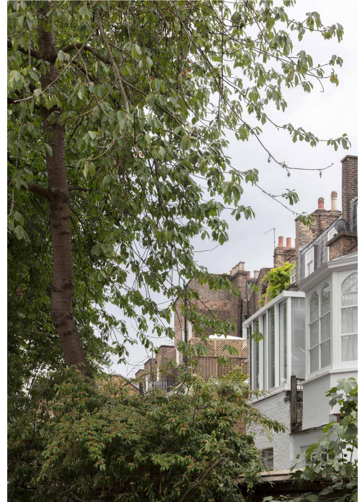
Rear outrigger extension to a listed building at Albion Street, Westminster by Architecture for London
