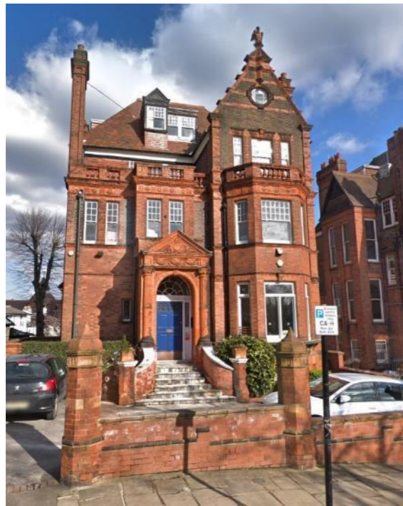
Figure 12: Grade II listed buildings on Lyndhurst Gardens (source: Google)
