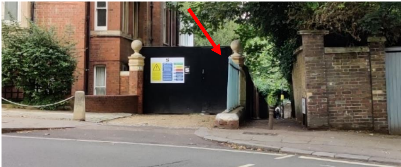
Figure 28: Boundary Wall viewed from Fitzjohn's Avenue (indicated with arrow), showing presumed 1970s extension at the front with stone finial, and the corresponding finial above the low curved wall de-marking the driveway entrance to 82 Fitzjohn's Avenue.
