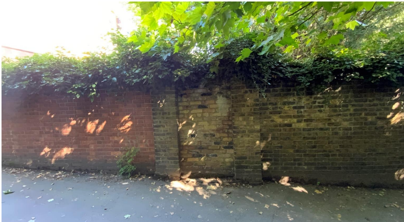
Figure 32: Point in the garden wall where the red brick meets the stock brick, and the location of a former gateway, now bricked-up. The replacement brick panel is in stretcher bond.
