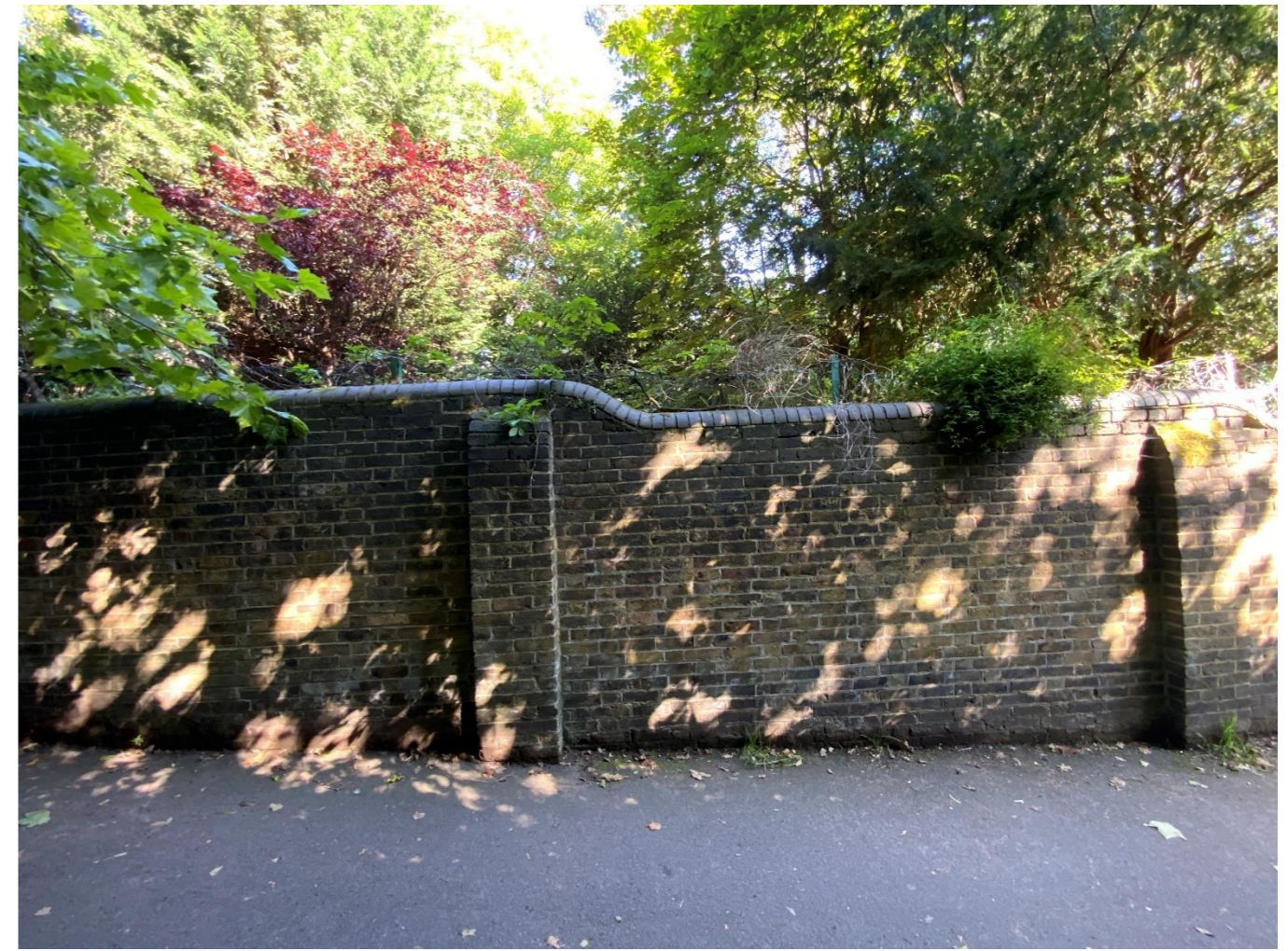
Figure 31: Area of the boundary wall that is thought to be more historic, constructed in stock brick in Monk bond with Staffordshire blue half round coping bricks.
