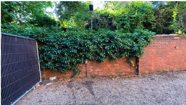
Image 02 - Section of the wall viewed from subject property
