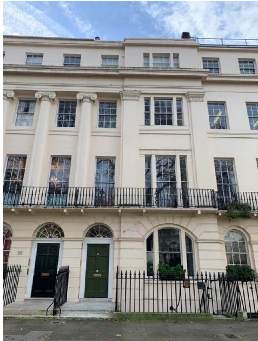
Entrance to Property from Fitzroy Square
