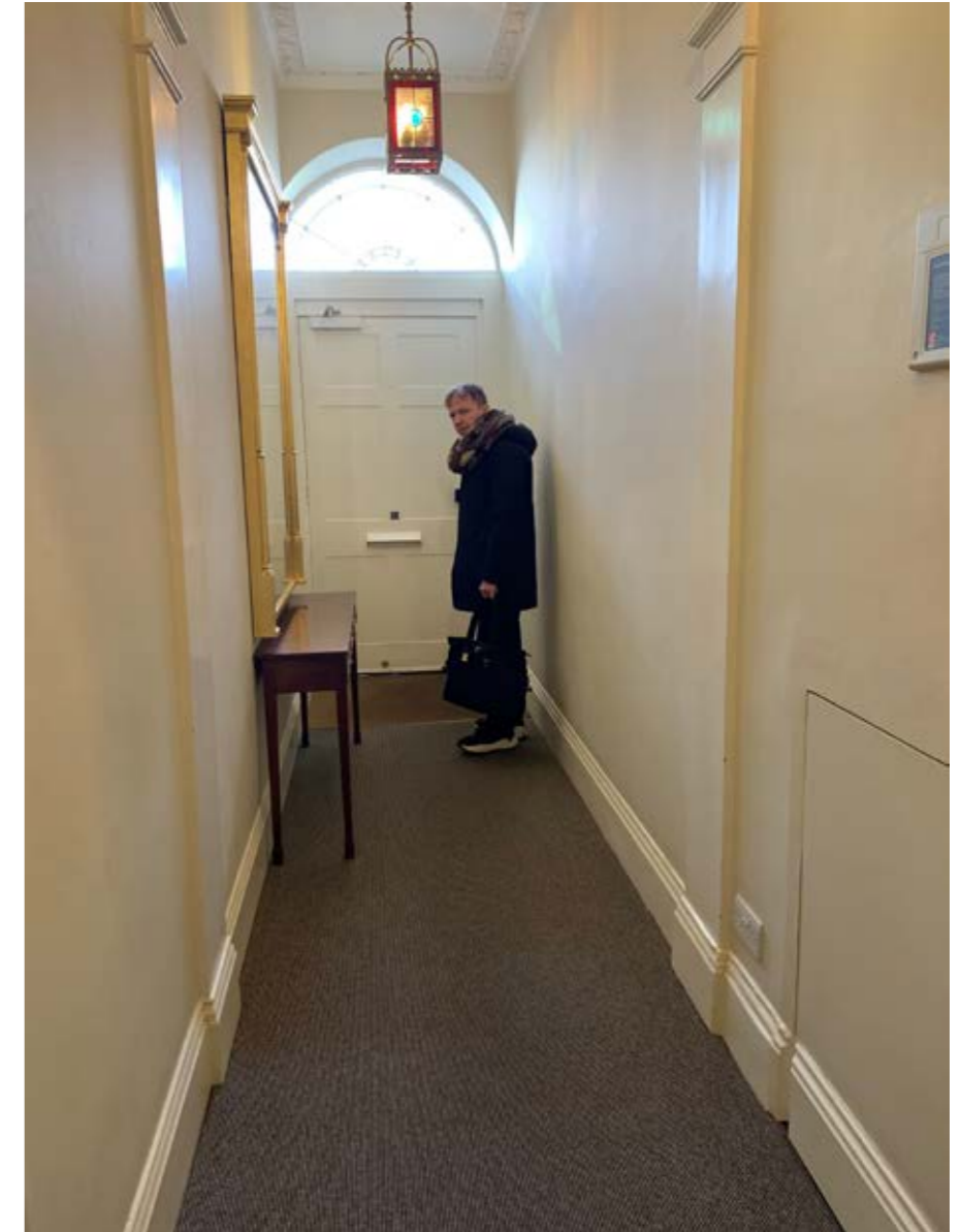
Entrance hallway at ground floor looking back towards entrance door
