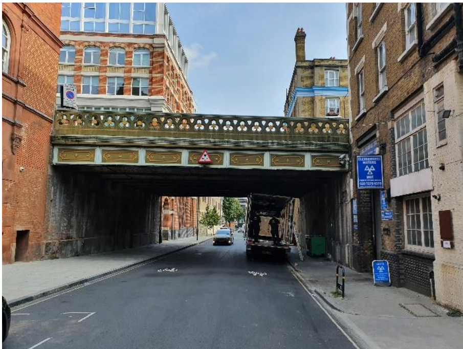
View from the property towards Warner Street showing the 14'3" restriction
